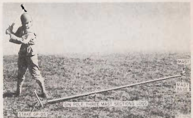
Figure 31. Driving Stake GP-25.
